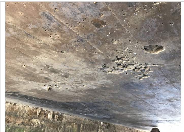
Span #2 has some minor honeycomb in the soffit area.
