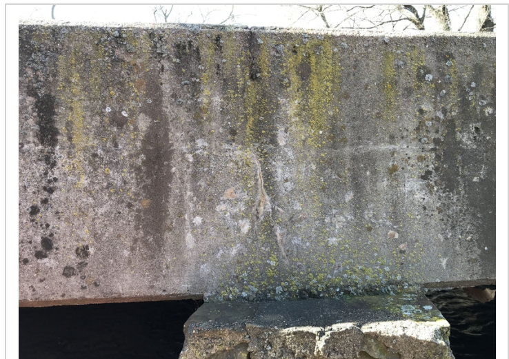
Vertical cracks in the side of the slab over pier #2 on both sides of the bridge.
