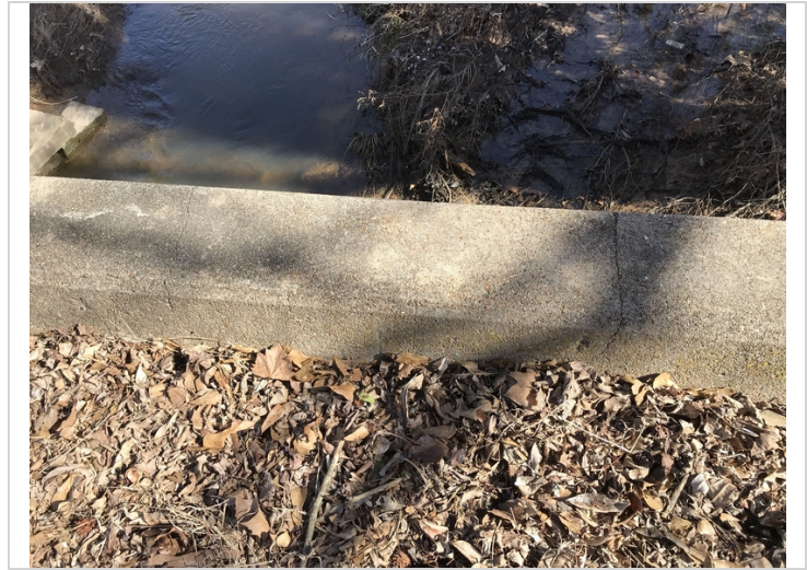
Both curbs have a few minor to moderate cracks in places.
