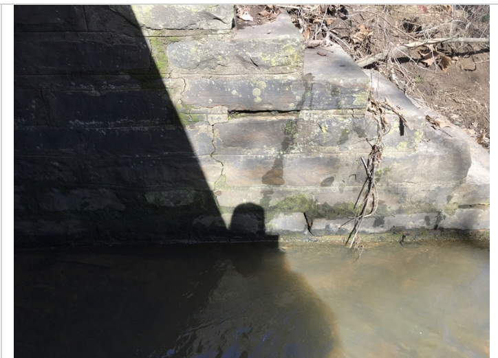
Abutment #3 has a few minor to moderate cracks in mortar joints in places throughout.
