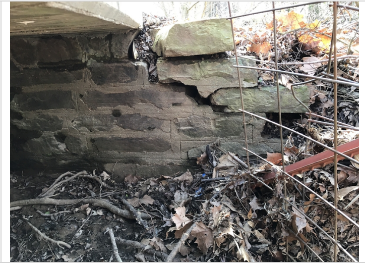
Abu#1 left side wing has a few masonry stones broken loose.
