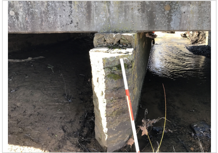
Pier #2 right end has a missing masonry stone from the top of the pier.
