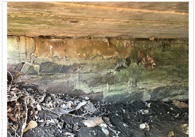
Abutment #1 has several minor to moderate cracks in the mortar joints in a few areas.
