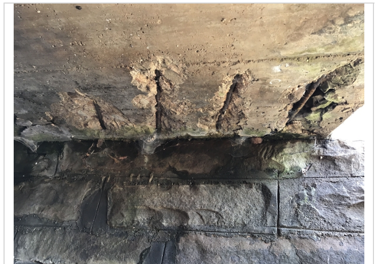
Span #2 right side at abutment #3 has some moderate spalls with exposed rebar in the soffit area.
