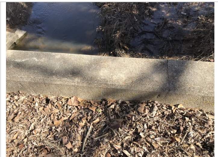
Dirt, leaves and debris are covering the deck drains.
